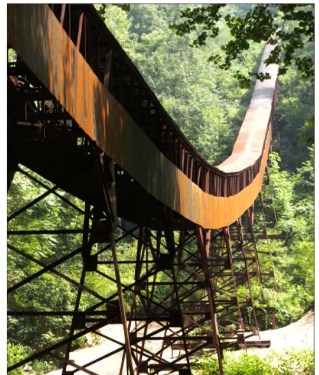
This coal conveyor, designed by Henry Ford, is still a dominant feature of Nuttallburg. National Park Service (JFB) photo.
